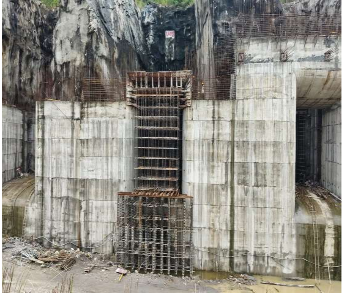
Vent 5 Bellmouth slab - Shuttering and alignment work in progress
